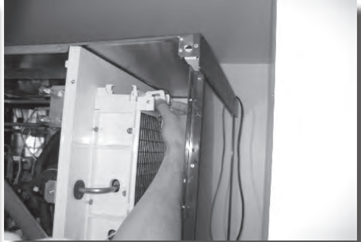
10. Remove and clean ice thickness sensor.
