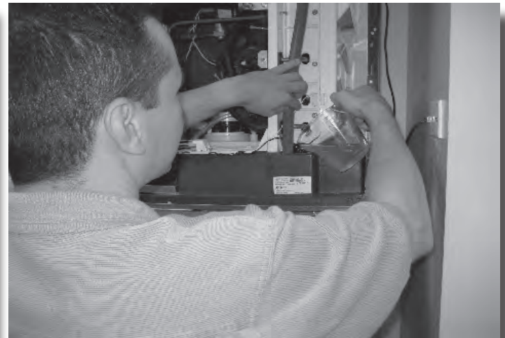
5. Wait until display code blinks 'A d 1', then add the scale remover.
