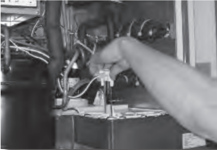
13. Remove and clean water level sensor.
